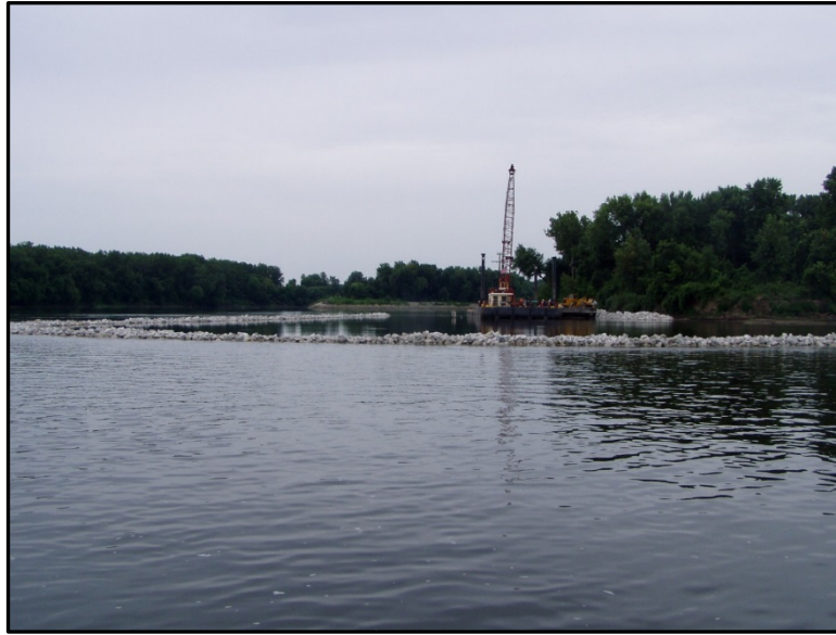
Photograph M-22: Chevron Construction (Gardner Division HREP 2005)
