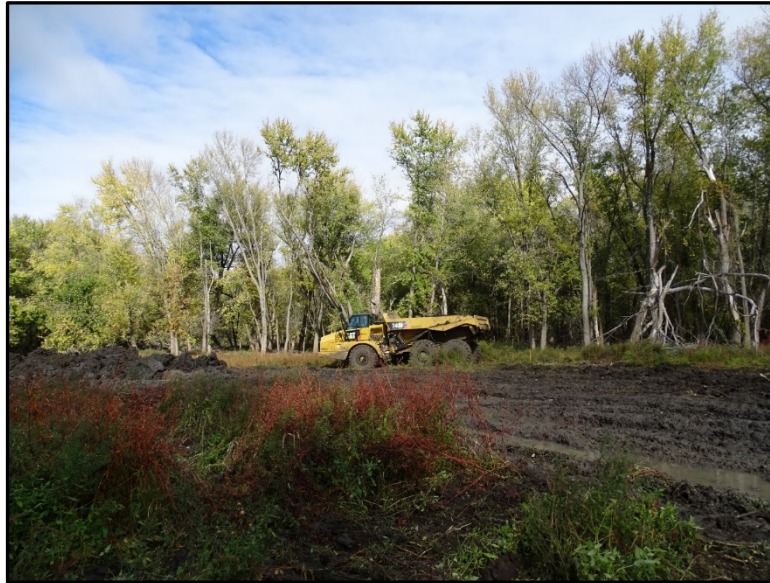
Photograph M-15: Huron Island HREP Stage I Transporting Excavated Material from Adjacent Placement Site to Forest Enhancement Site
