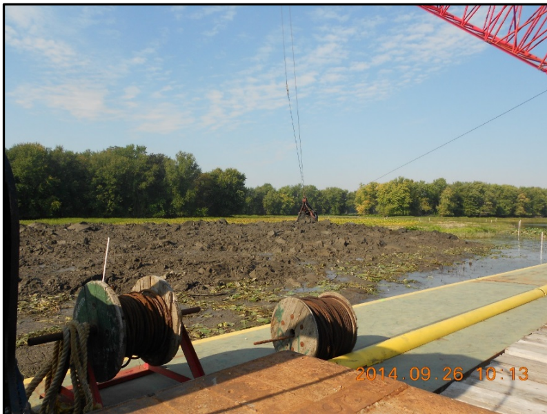
Photograph M-5: Pool 12 Overwintering HREP Stage I Bucket on Crane
