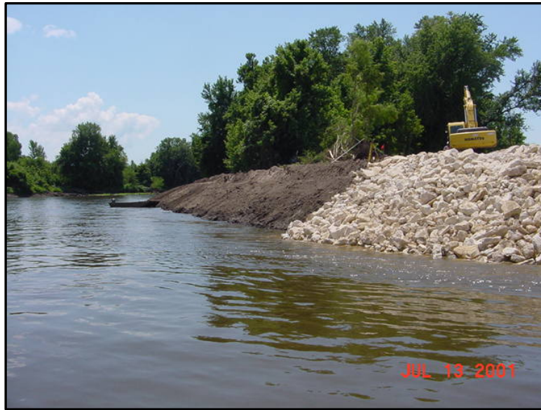
Photograph M-25: Rock Placement Following Shaping (Gardner Division HREP)
