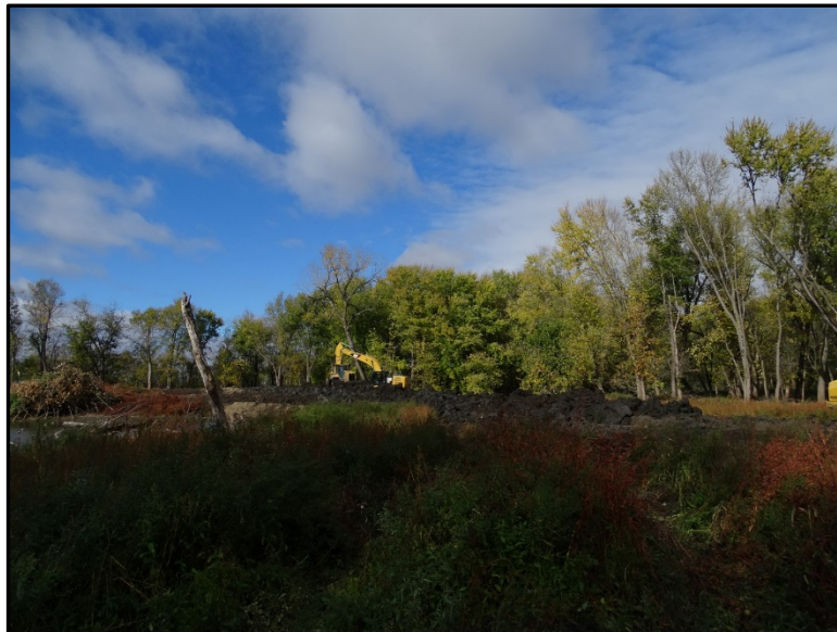
Photograph M-16: Huron Island HREP Stage I Shaping Material Transported to Forest Diversity Site
