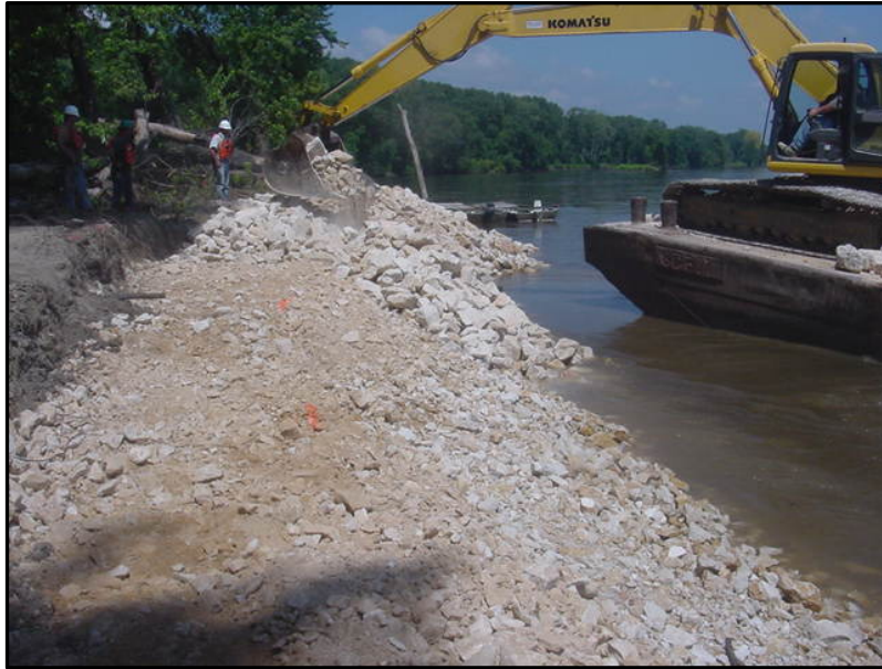
Photograph M-27: Riprap on Bedding Stone (Shot Rock) at Gardner Division HREP
