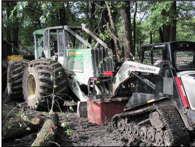
Photograph M-11: Tree Clearing Equipment (Huron Island HREP)
