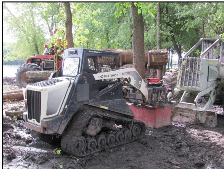
Photograph M-10: Tree Clearing Equipment (Huron Island HREP)
