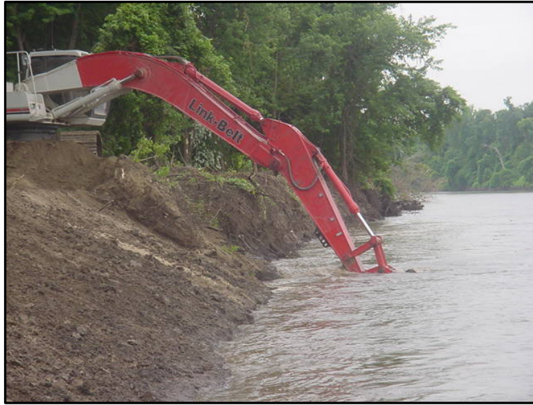
Photograph M-23: Bankline Shaping Prior to Receiving Rock Protection (Gardner Division HREP)
