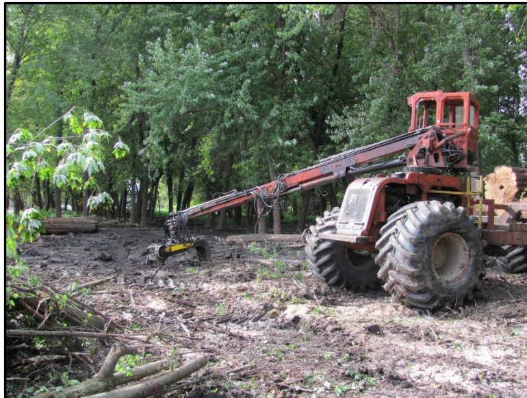
Photograph M-12: Tree Clearing Equipment (Huron Island HREP)
