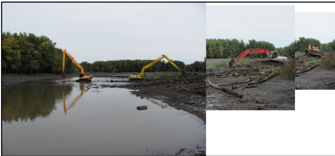
Photograph M-7: Partially Drained Pool with Excavators (Huron Island HREP Stage I)
