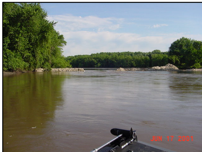
Photograph M-21: Notched Closure Structure (Gardner Division HREP)
