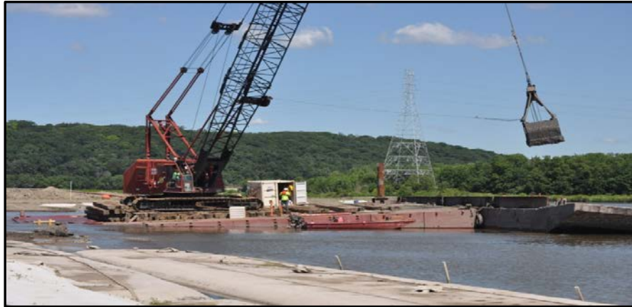
Photograph M-6: Barge-mounted Crane with Clamshell Bucket (Peoria Islands)
