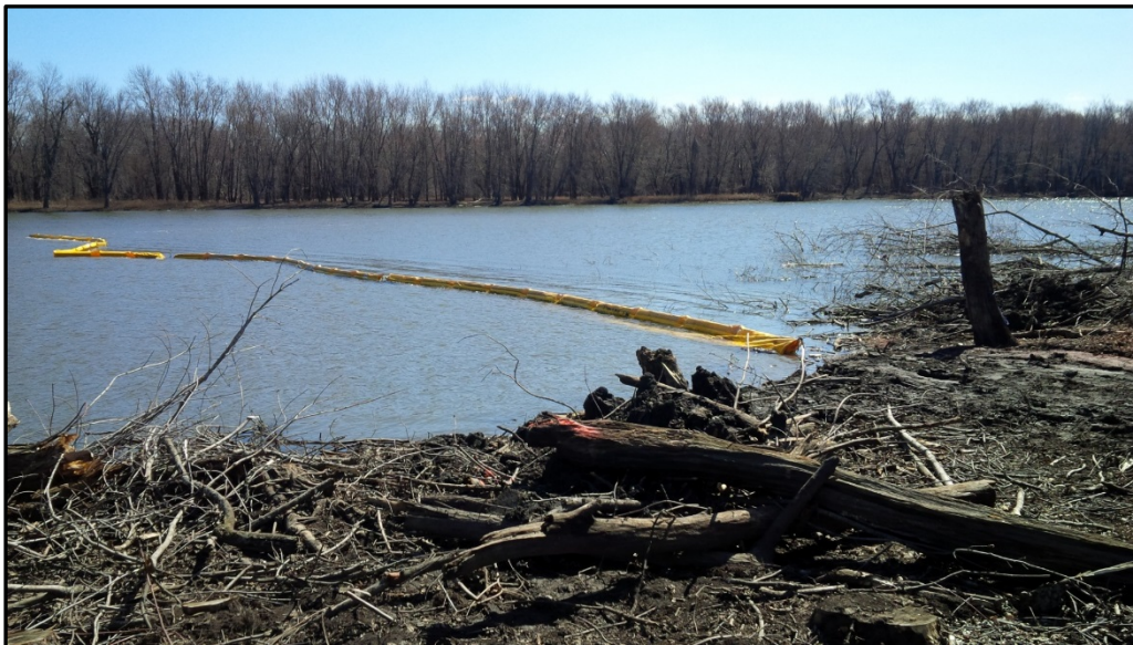
Photograph M-1: Turbidity Curtain (Huron Island HREP Stage I)
