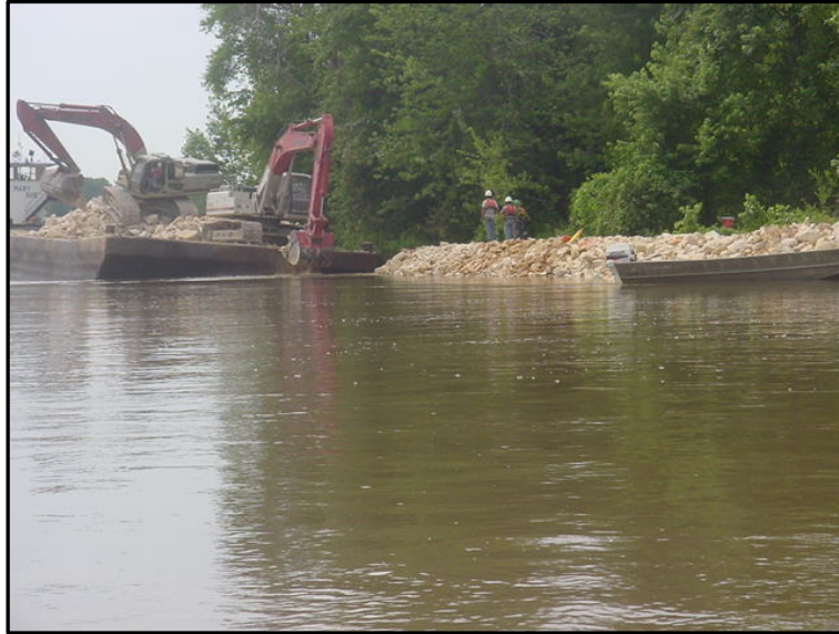
Photograph M-26: Transporting Rock from Barge to Bankline (Gardner Division HREP)
