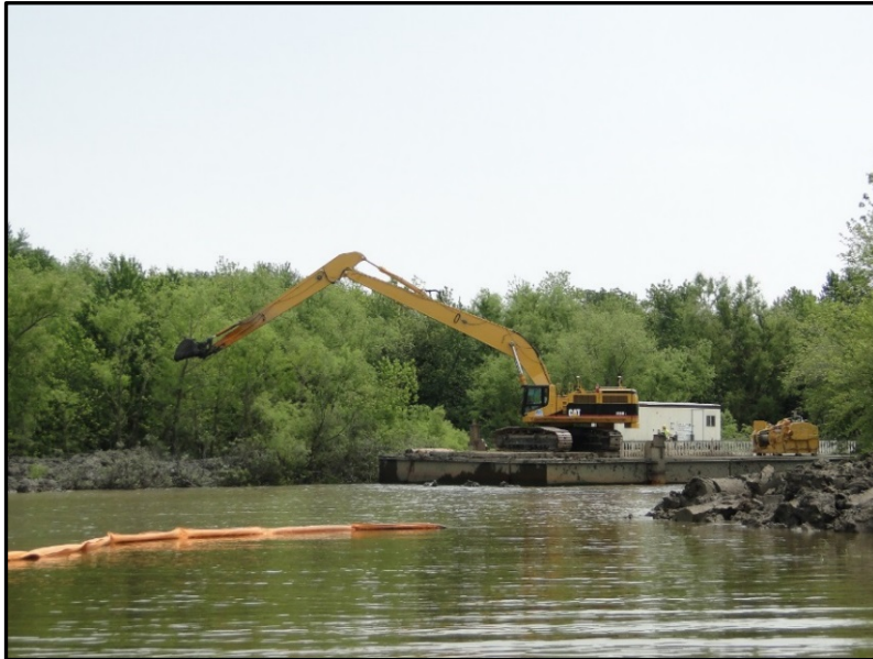
Photograph M-4 Lake Odessa HREP Stage IIB Barge Mounted Excavator
