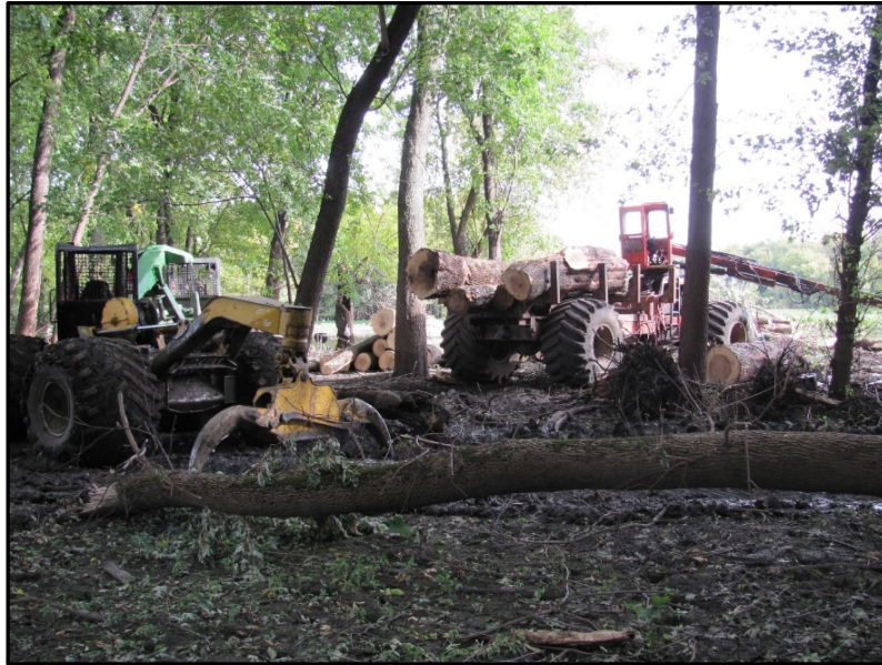
Photograph M-9: Tree Clearing Equipment (Huron Island HREP)
