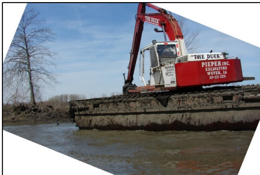
Photograph M-3: Floating Excavator (Lake Odessa HREP)
